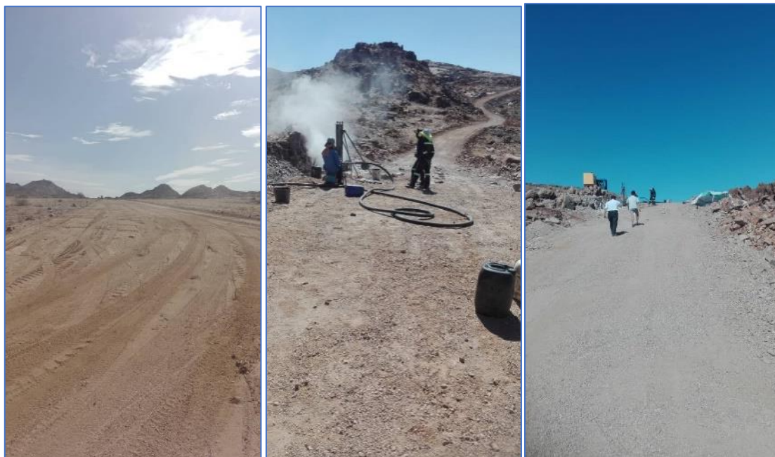
Figure 1 – Completed road between nearest traversable road to Swanson Plant
